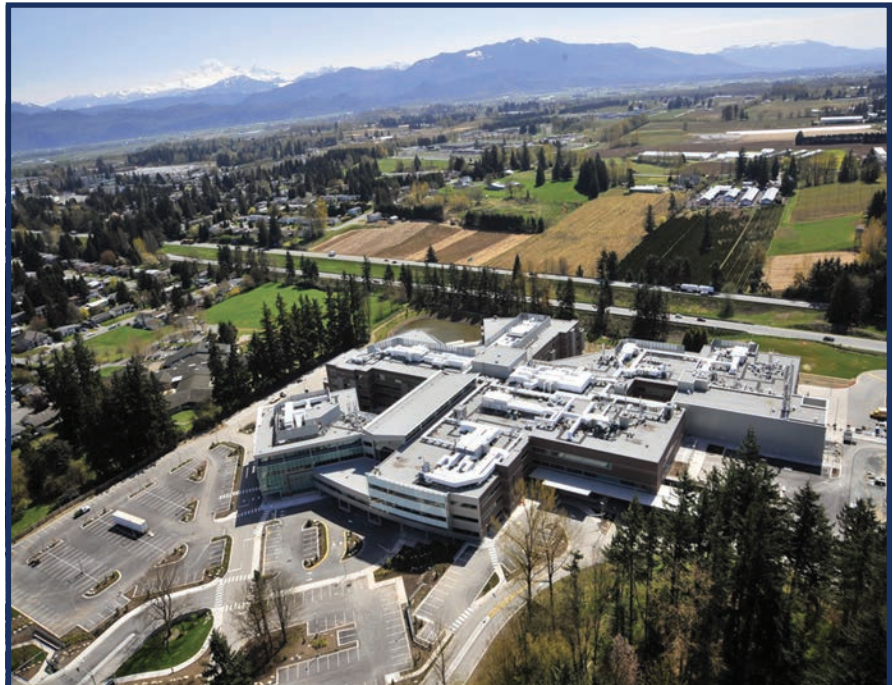
The hospital uses less than half the energy used in the industry average.
