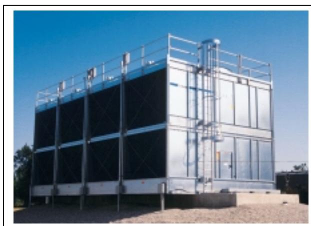
Forced draft towers have fans on the air inlet to push air either counterflow or crossflow to the movement of the water. Forward curved fans are often employed. They use more fan power than induced draft but can provide external static pressure when required. This can be important if the cooling tower requires ducting, discharge cap or other device that creates a pressure drop.
